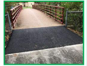
Briar Creek Park bridge 2024
