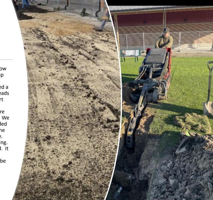
I was able to borrow a trencher to finish up some work on the driving range. Lalo led a project to install 3 heads between the new cart barn and range tee. Pipe and 3 heads were installed and tested. We also graded and seeded the area to expand the back of the range tee. All 3 heads are working. The seed germinated. It will take a couple months to fill in and be playable.
