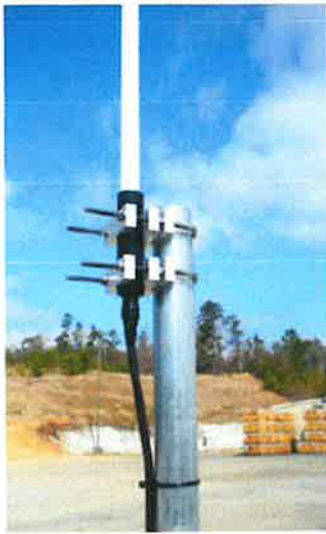
Figure 84 – RF Antenna to Mast
